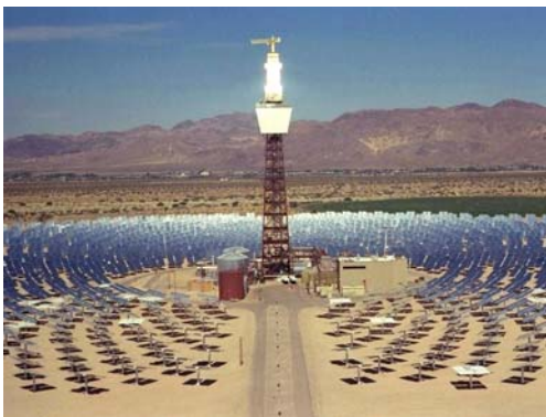
Solar Tower, Barstow, California
