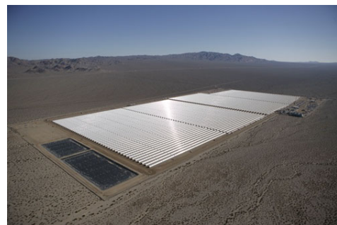
Nevada Solar 1, Las Vegas a 64 Megawatt parabolic trough system.
